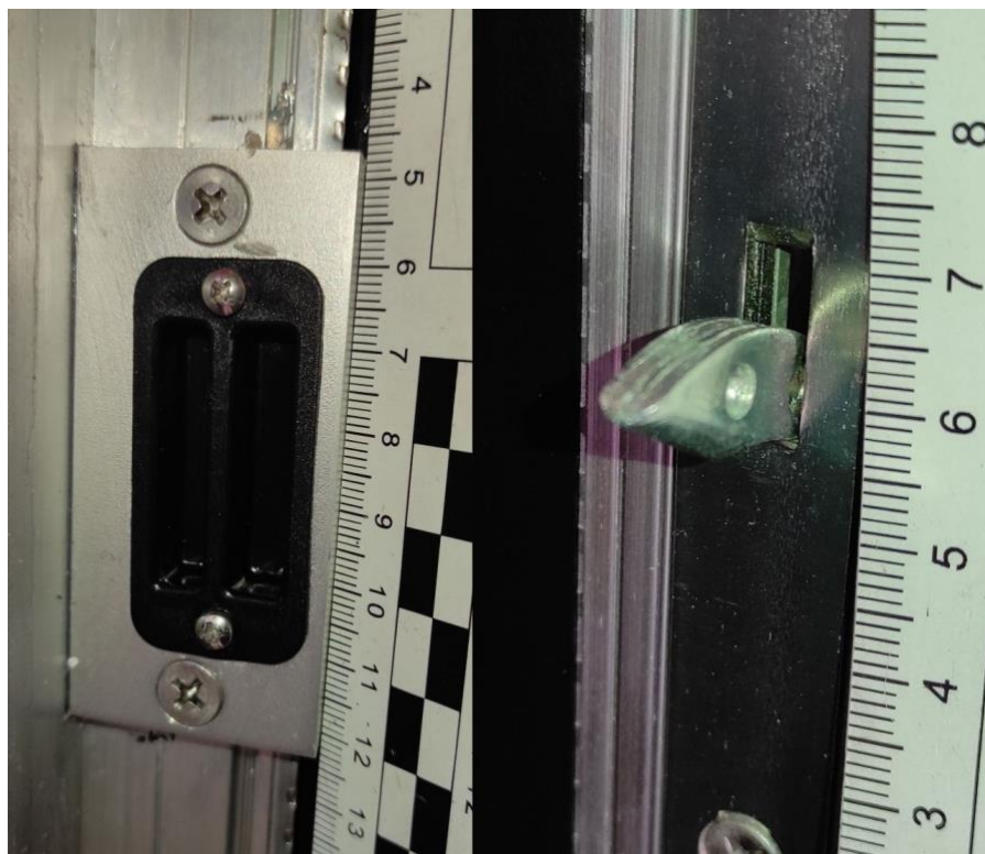
Locking components in frame and sash.
